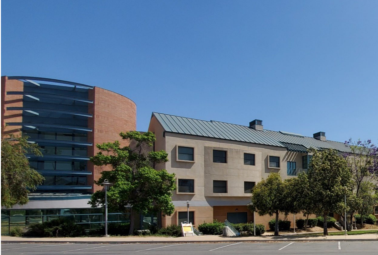
Photograph 3. Pentland Hills Residence Halls
