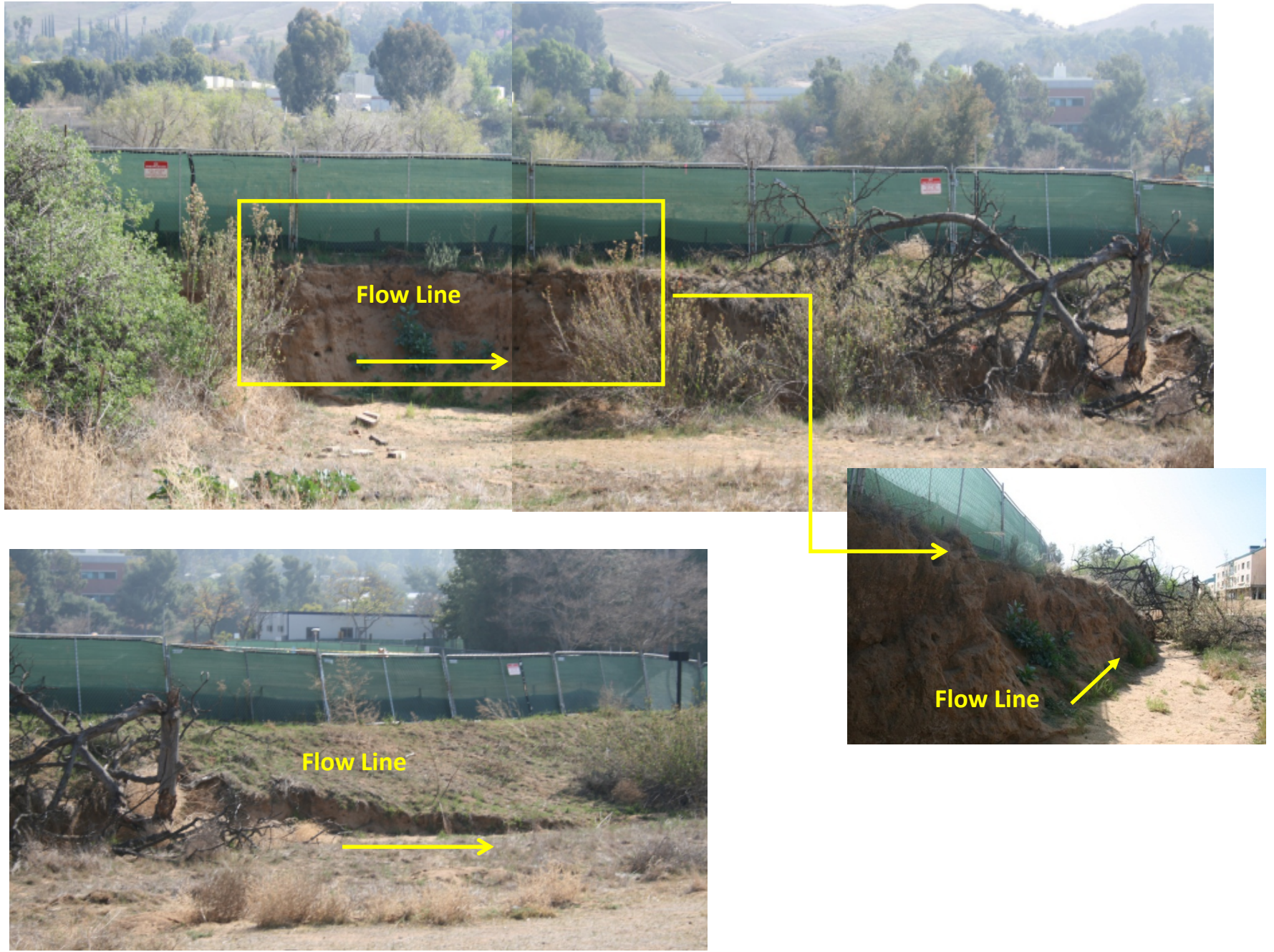
Figure 2: Reach 1 - Existing Arroyo Site Conditions
