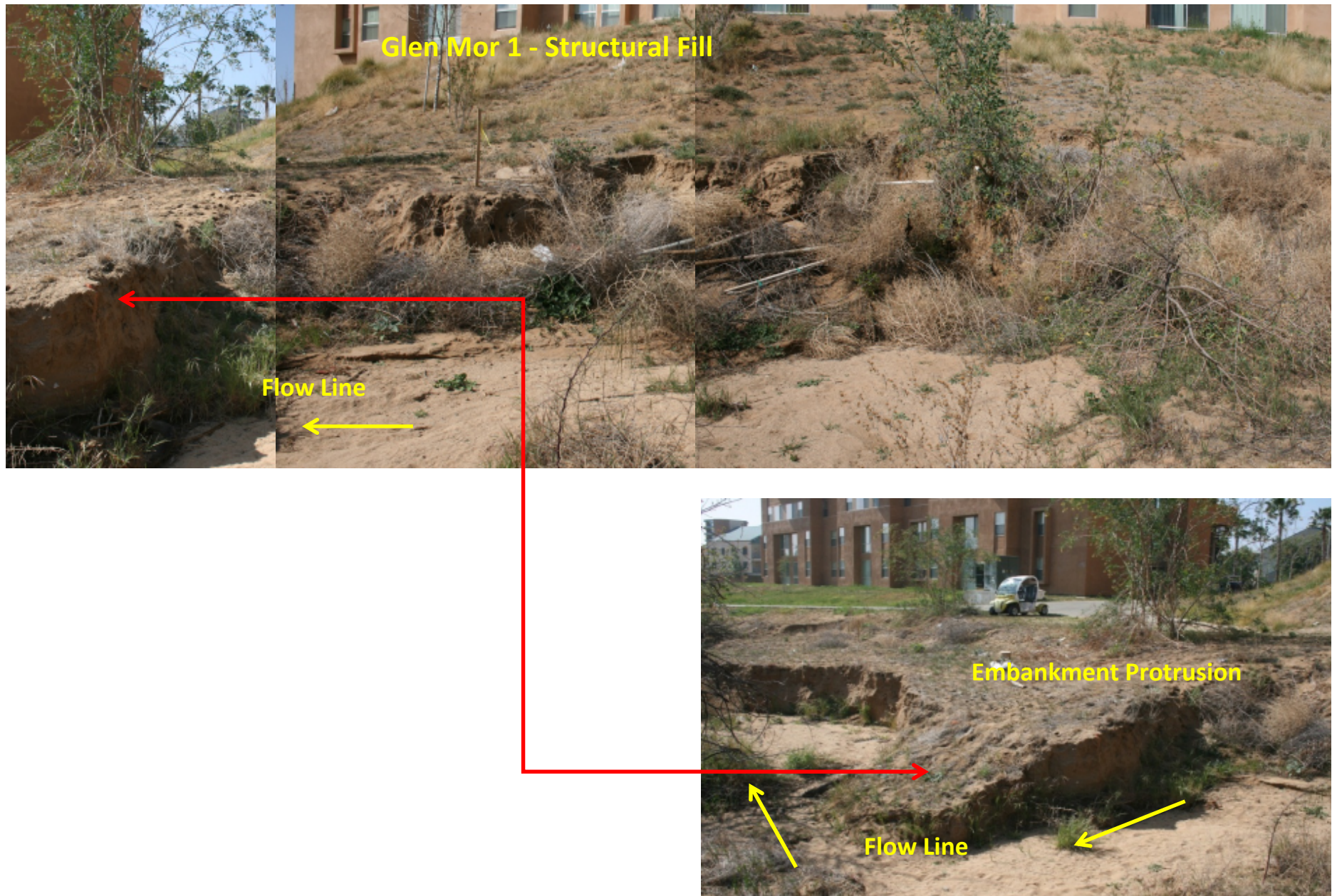
Figure 5: Reach 2 - Bend 3 Existing Arroyo Site Conditions and Glen Mor 1 Structural Fill Scarp
