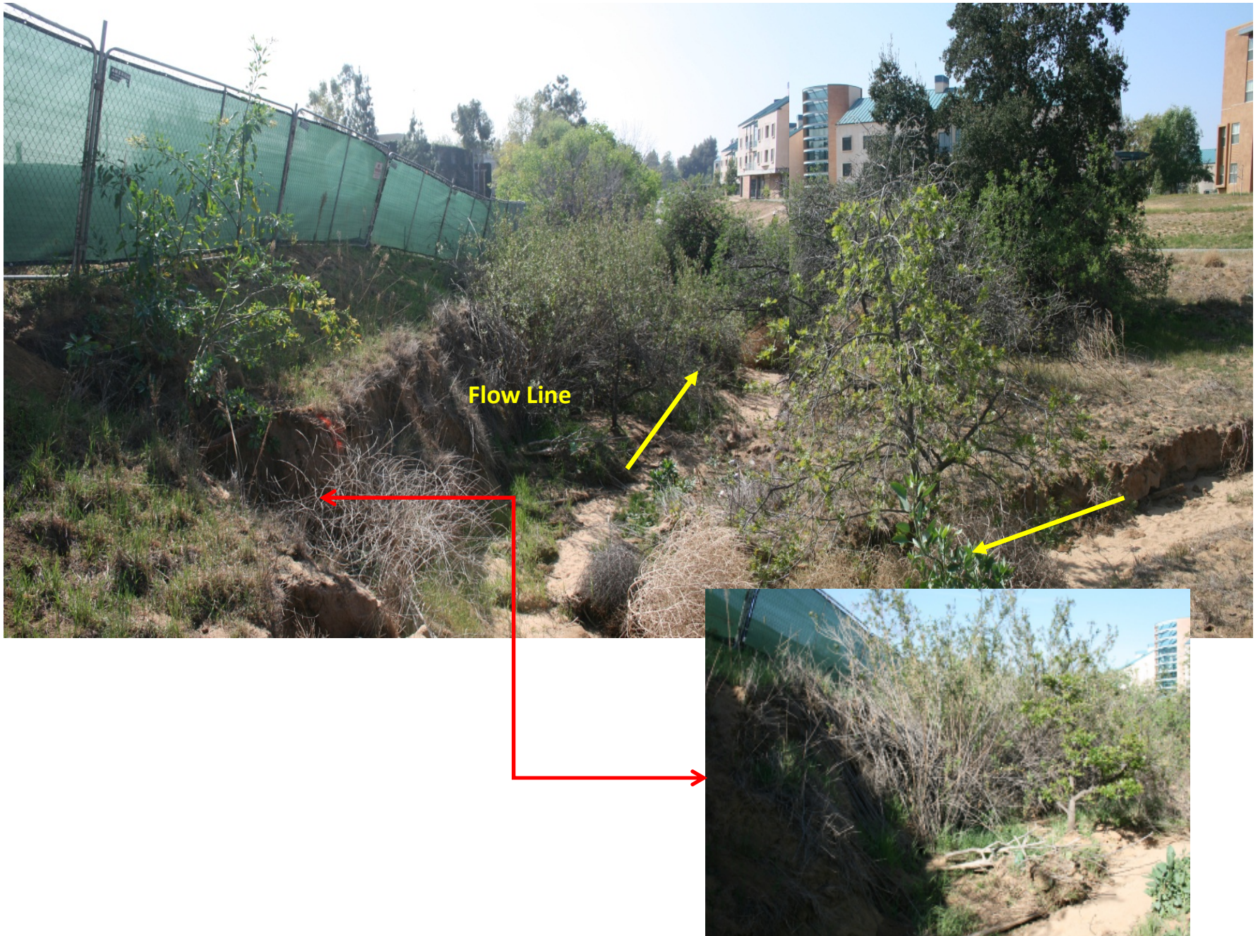
Figure 3: Reach 1 - Existing Conditions 90 Degree Angle of Attack at Slope Scarp
